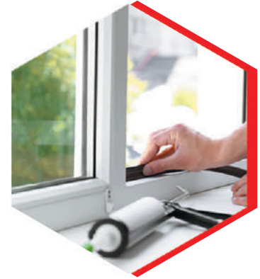
Glazing Repairs & Installations
