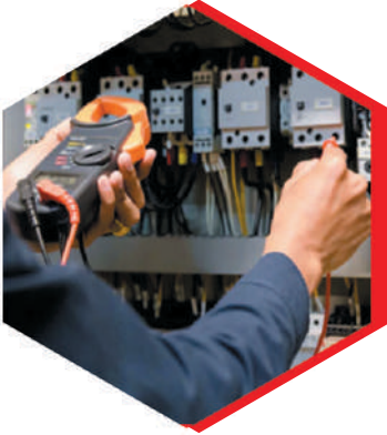
Mechanical & Electrical Maintenance
